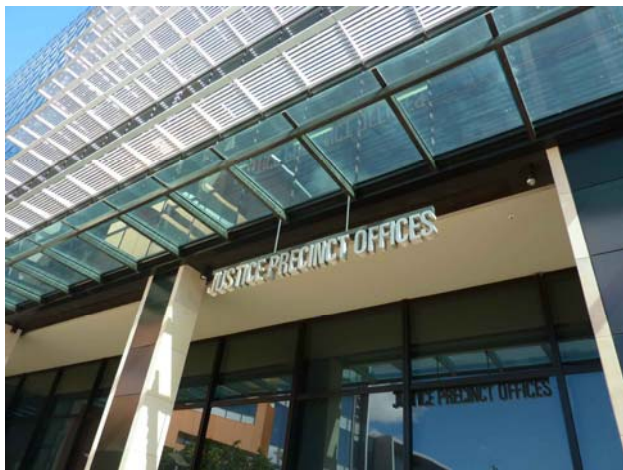
(FFMPU's offices, Parramatta)
